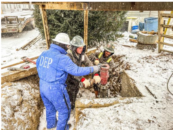
Bear Run 001 Plugging February 2023
