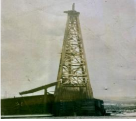
Drilling the A. Lorenzen #15 – August 1927
