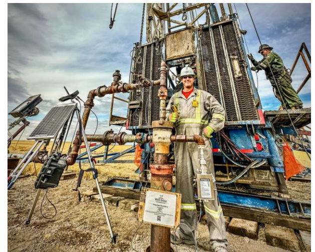
Plugging Crew October 2023
